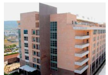
Sand stone cladding of external façade to minimise heat impact
